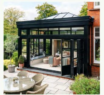
offering a smooth connection to the beautiful gardens beyond. To achieve this, a steel frame was bolted into the new foundation, providing the necessary strength and stability, while a timber subframe was used to create openings for the windows, doors, and the glazed Lantern.
