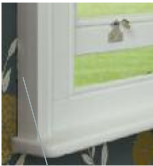
Normal Replacement Box Sash may project into the room.
